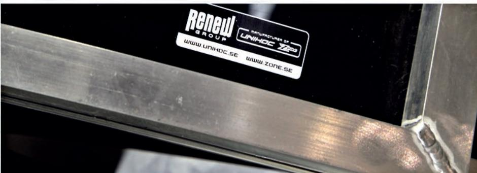
The new rink has been created in full compliance with the standards of the European REACH law. The REACH regulation is a law that ensures that products within the EU do not contain any prohibited or dangerous chemicals. The plastic parts are made of thick 6 mm PP plastic which has long durability and the frame is made of high quality aluminum.
